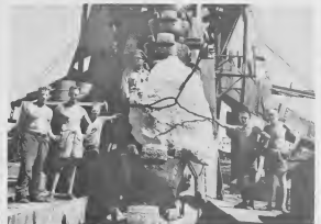
WHILE DREDGING in the vicinity of No. 3 Finger Pier's north basin, the dredge had a tussle with this man-dwarfing chunk of coral. MIENTRAS E tabata draga den vecindario di e basin di nord di No. 3 Finger Pier, e draga mester a lucha cu e pida baranca grandi aki.
